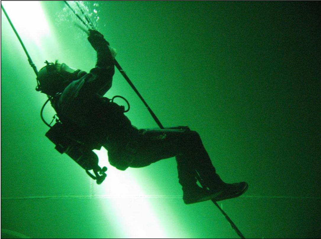
*Figure 4: Diver secures the control tables to the stainless steel guide wire using zip ties.*
