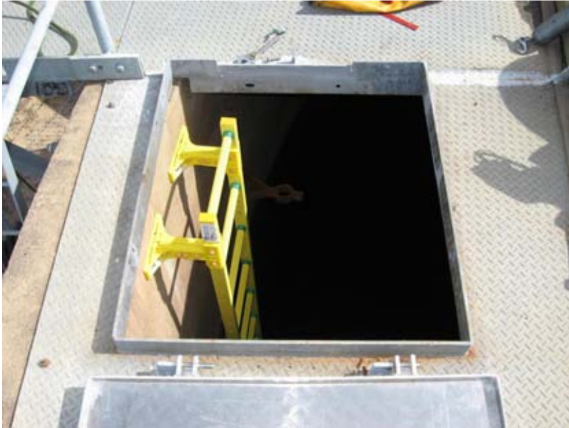
Figure 3: The hatch frame sealed off and a new vertical ladder fitted.
