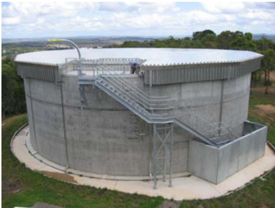
Figure 1: An impressive external stairway but the entry hatch and platform areas remain unsealed.
